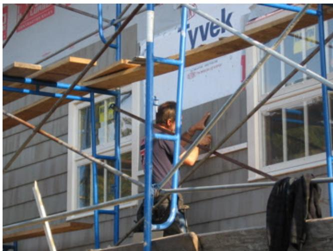
Our contractor, Thoughtforms Corp., has made excellent progress on the barn renovation. The structure is stabilized, the new windows are in, and thick insulation is being installed on the walls. The last steps of this phase will be completed in November: red cedar siding, the newly installed roof, and painting.
